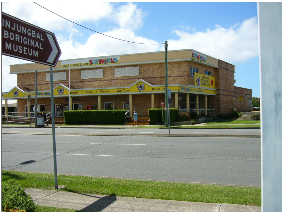
Figure 5: view east over 34-38 Minjungbal Drive
