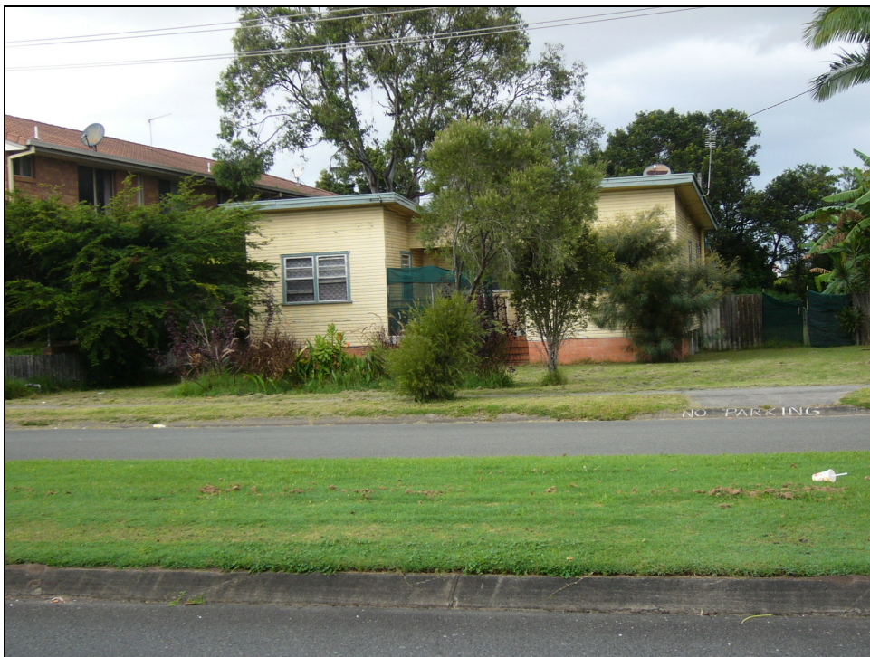
Figure 9: View south 52 Kirkwood Road East
